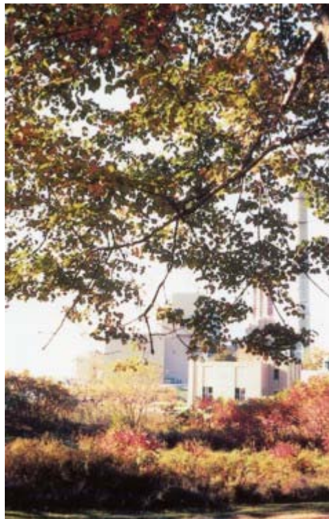
Power Plant New England Coast, Massachusetts
