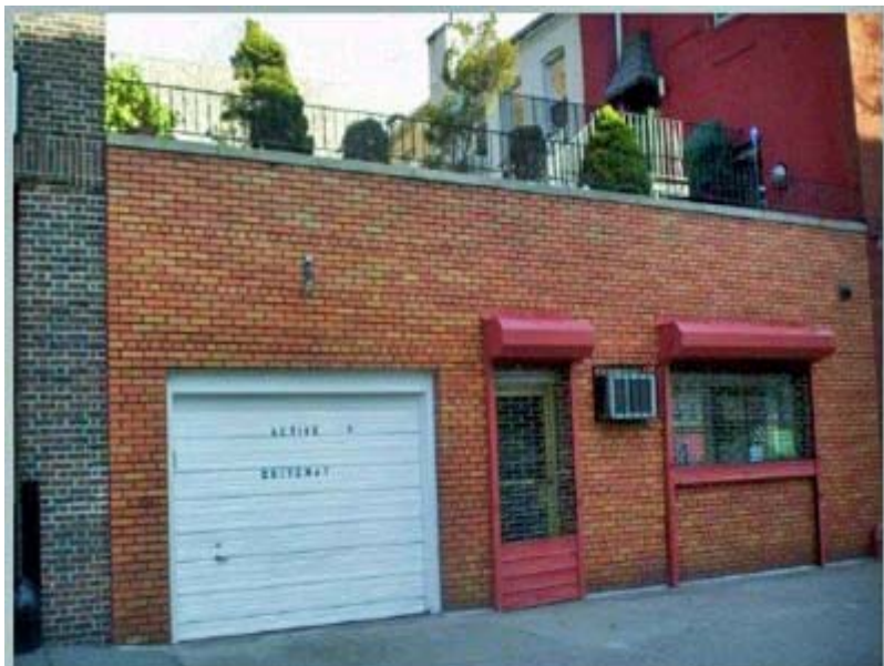
This recently converted sales office was once an active print shop.
