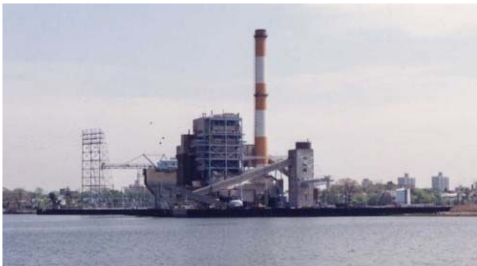
Typical Northeast Power Plant
