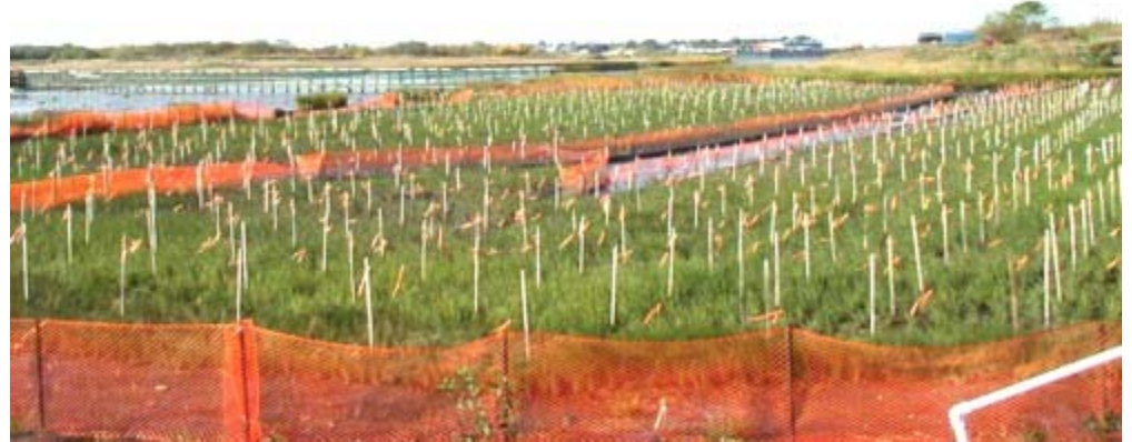
Nearshore tidal plantings, wildfowl exclusion barrier in place
