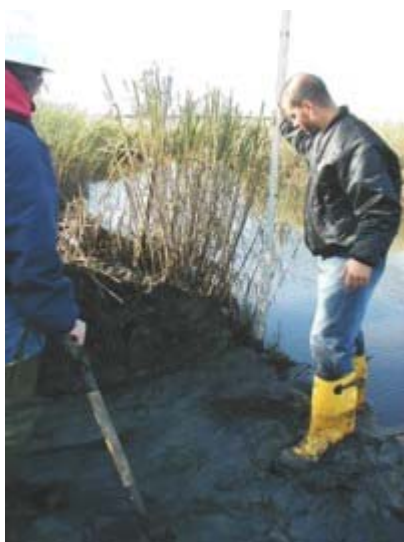
Elevations are repeatedly taken when crafting tidal wetlands
