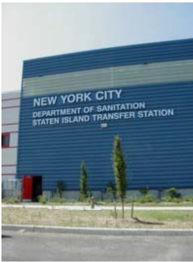
Transfer Facility Building is complete
