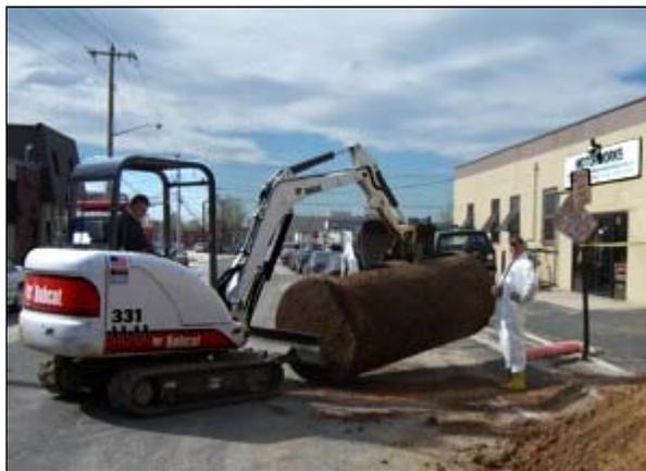
*Removal of Leaking Underground Petroleum Tanks*
