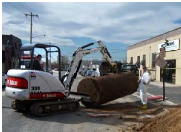
Removal of Leaking Underground Petroleum Tanks
