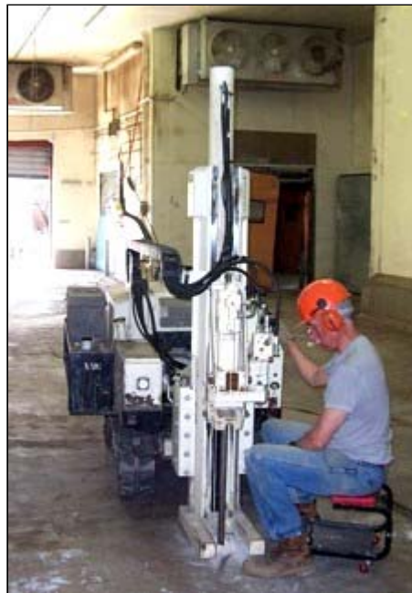
Subsurface Testing inside Building using a Track-mounted Geoprobe
