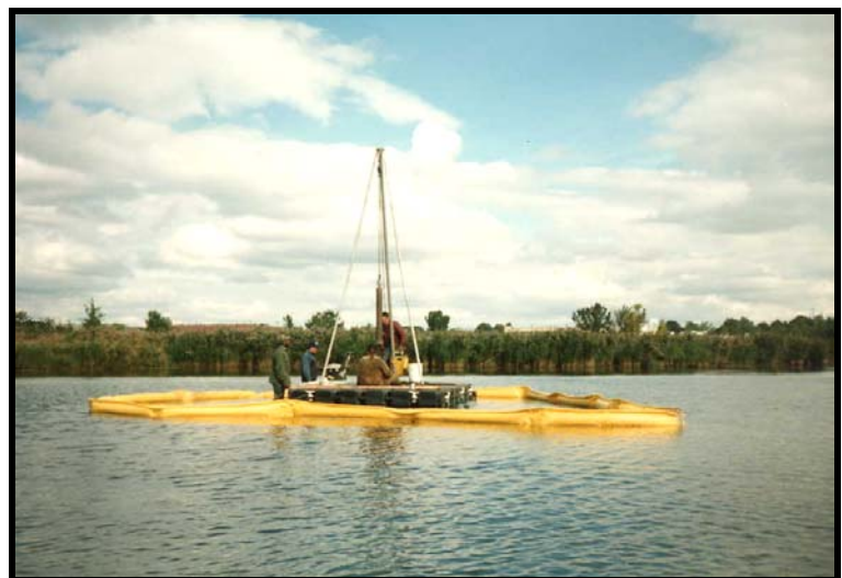
Phase II Testing of Former Runway at Flushing Airport
